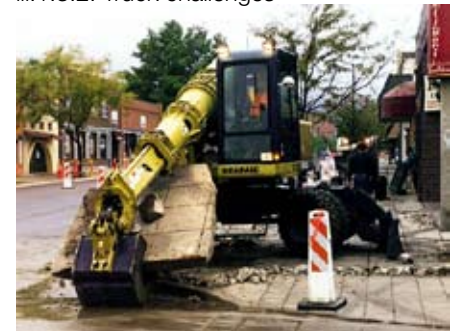
ill. 1.3.3: Gradall excavator
