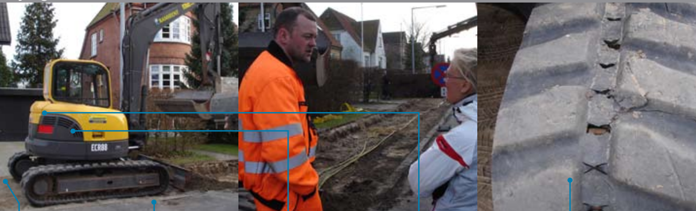
Laying cables Kjærlundsvej in Aalborg inner city Functions: Digging trenches
